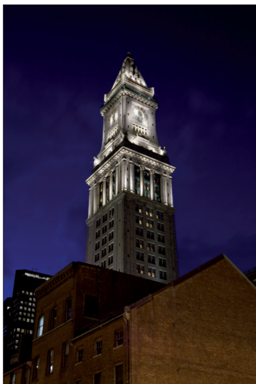
Obr. 2. Marriot Custom House Tower – detail
