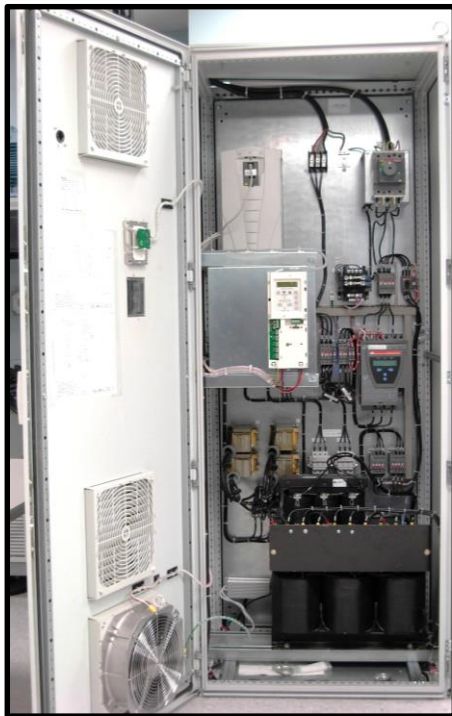
20 HP, 18-pulse package with soft-start bypass
