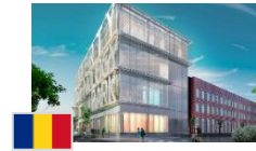
Liberty Technology Park, Cluj , Rumunsko
