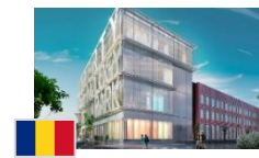
Liberty Technology Park, Cluj , Rumunsko
