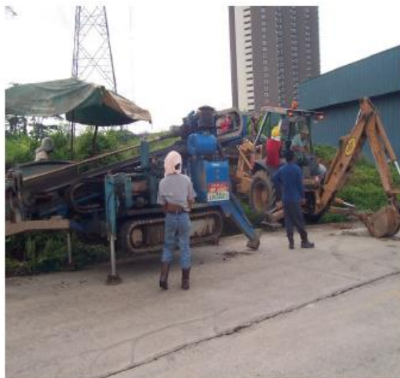
Excavator (3 rd party digging)
